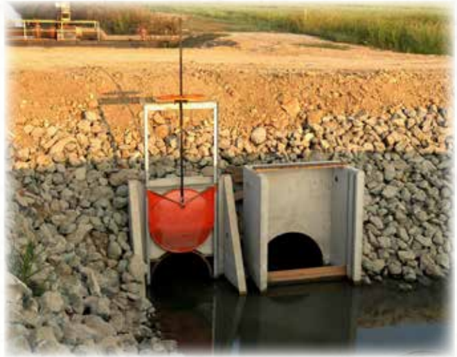
This water management structure was installed as part of the Montna Farms’ RCPP practices to facilitate more efficient water use.
